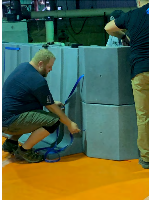
Figure 13. Crew installing the top 90° corner unit.
