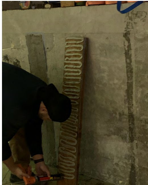
Figure 11. Installation of support boards in the wingwall.
