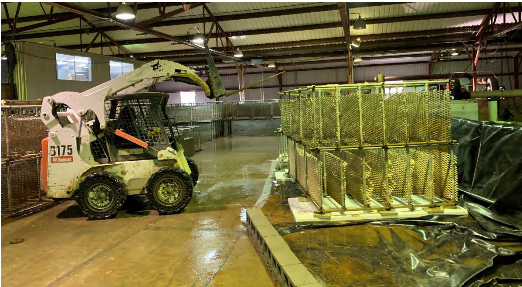
Figure 47. Placement of additional metal frames to hold down the guide vane.
