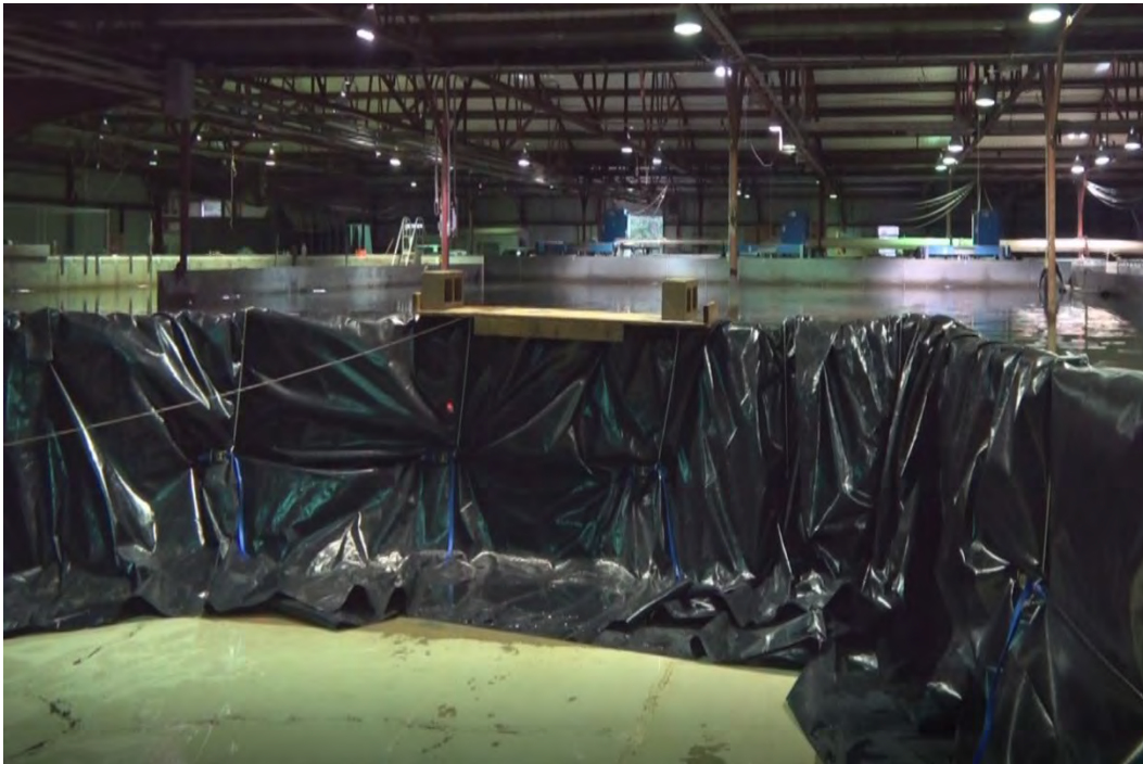
Figure 43. Plywood setup for liner cover protection at center wall.
