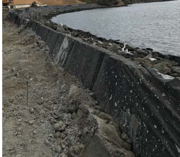
Figure 4: Muscle Wall as a liquid waste containment barrier
