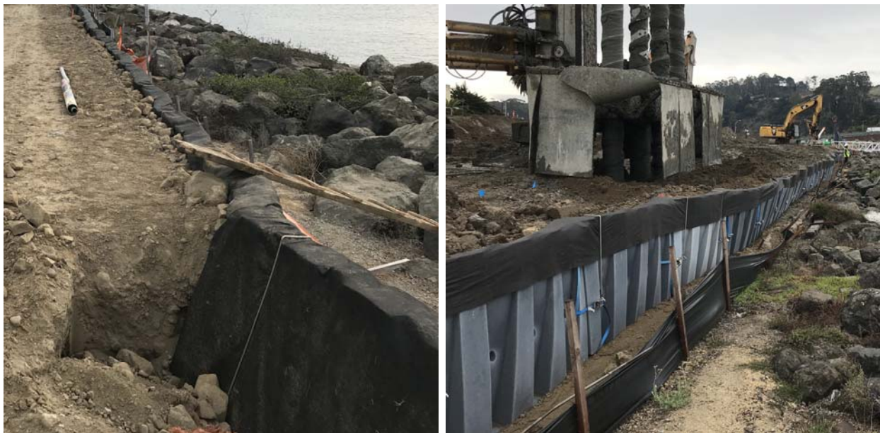
Figure 3: Muscle Wall acting as a temporary retaining wall for soil
